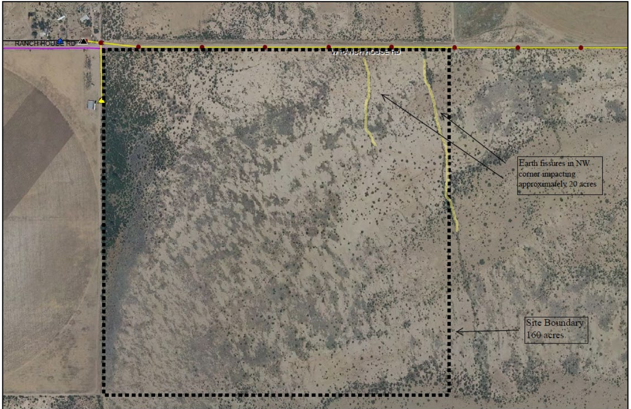
Ranch House Solar Site
