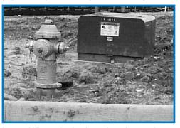
line as a fire hydrant. When designing electric service to a new subdivision, it is advisable to review the construction drawings of the water system to identify the proposed locations of fire hydrants prior to designing the electric service. If an existing transformer is to be replaced that is in close proximity to a fire hydrant, the designer should check the applicability of this new rule.
